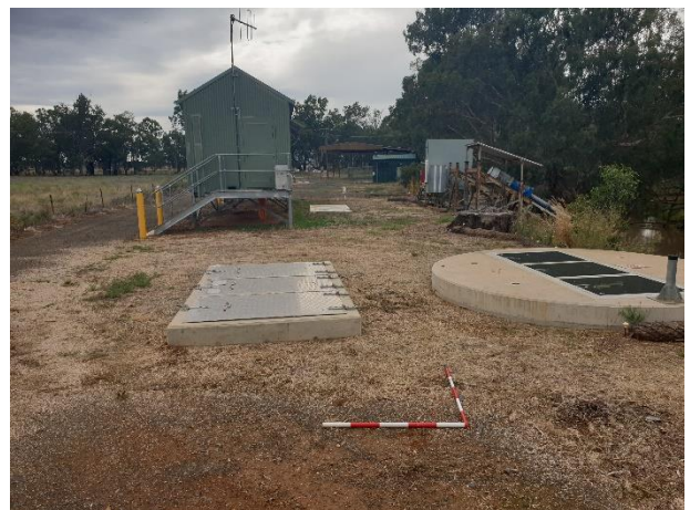
Figure 5-10: View east of disturbances from the construction of existing pumping station
