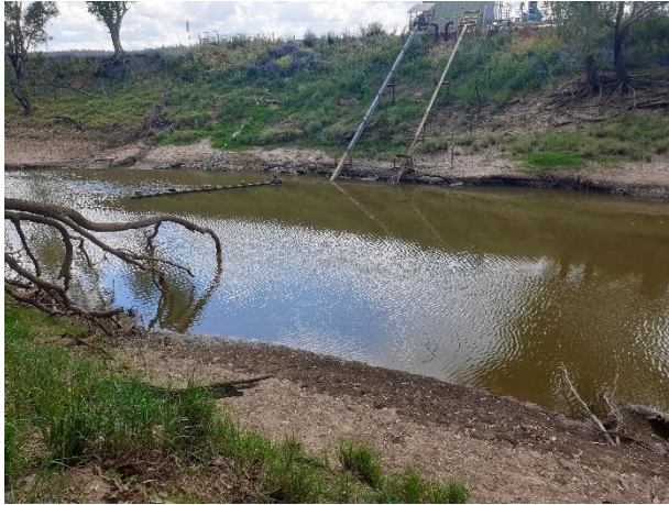
Figure 5-5: View north of existing pump station on the Lachlan River
