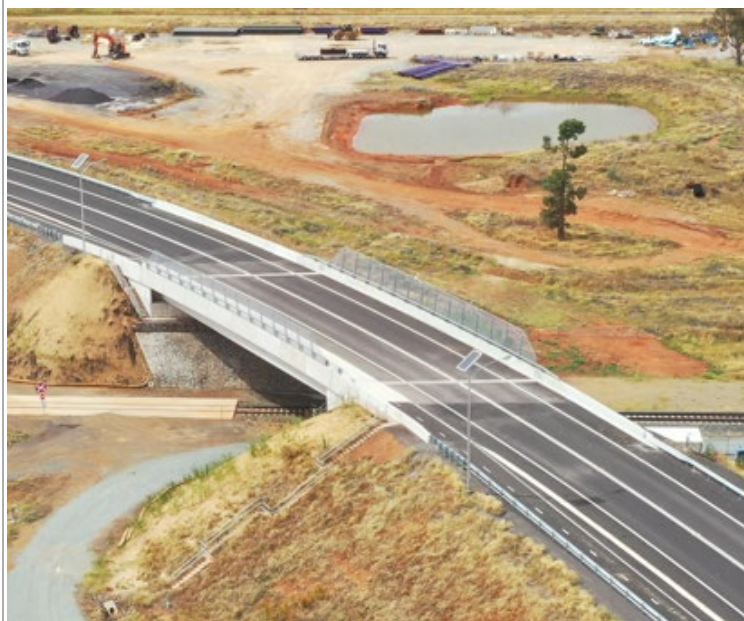
Yvonne Hutton Bridge
