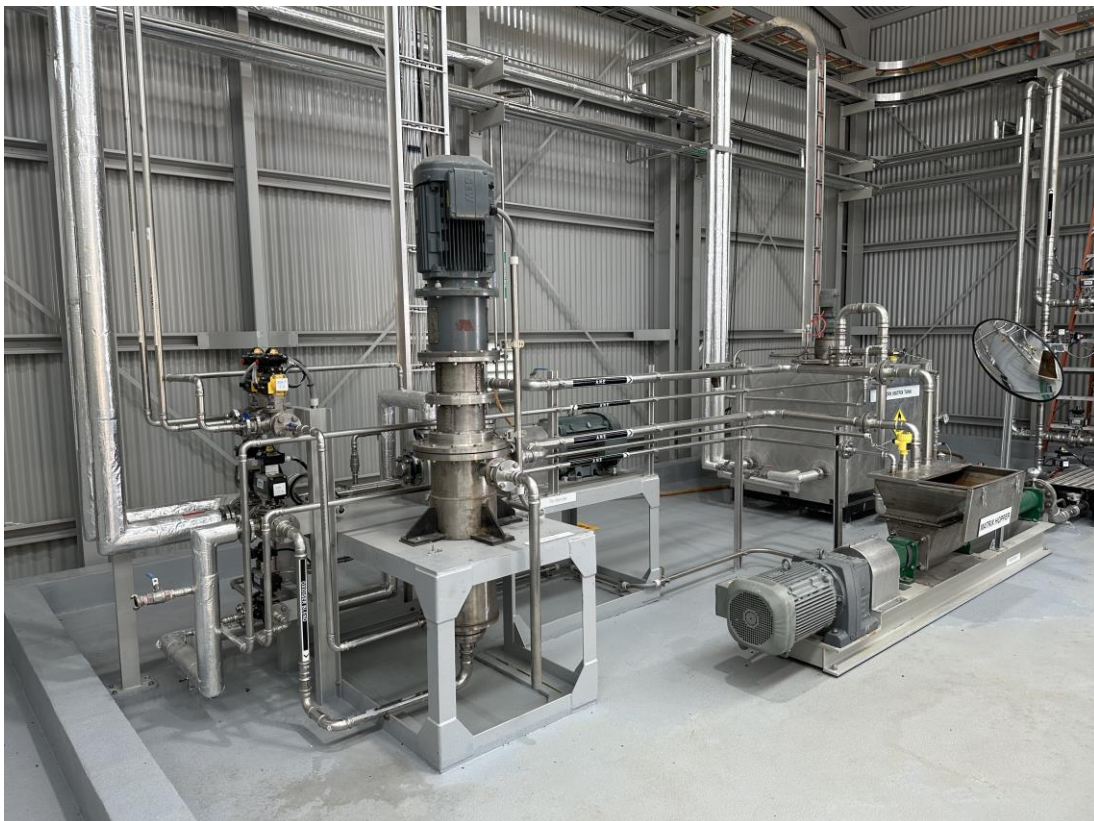
Figure 7: Emulsion Blender, Hopper, and Rework Tank
