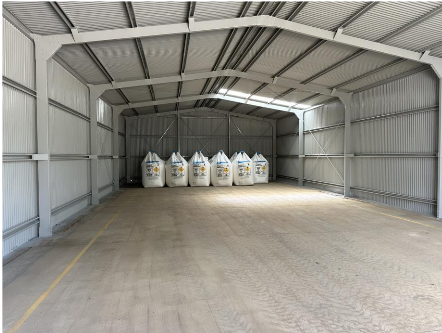
Figure 4: Storage of AN bags in the Shed
