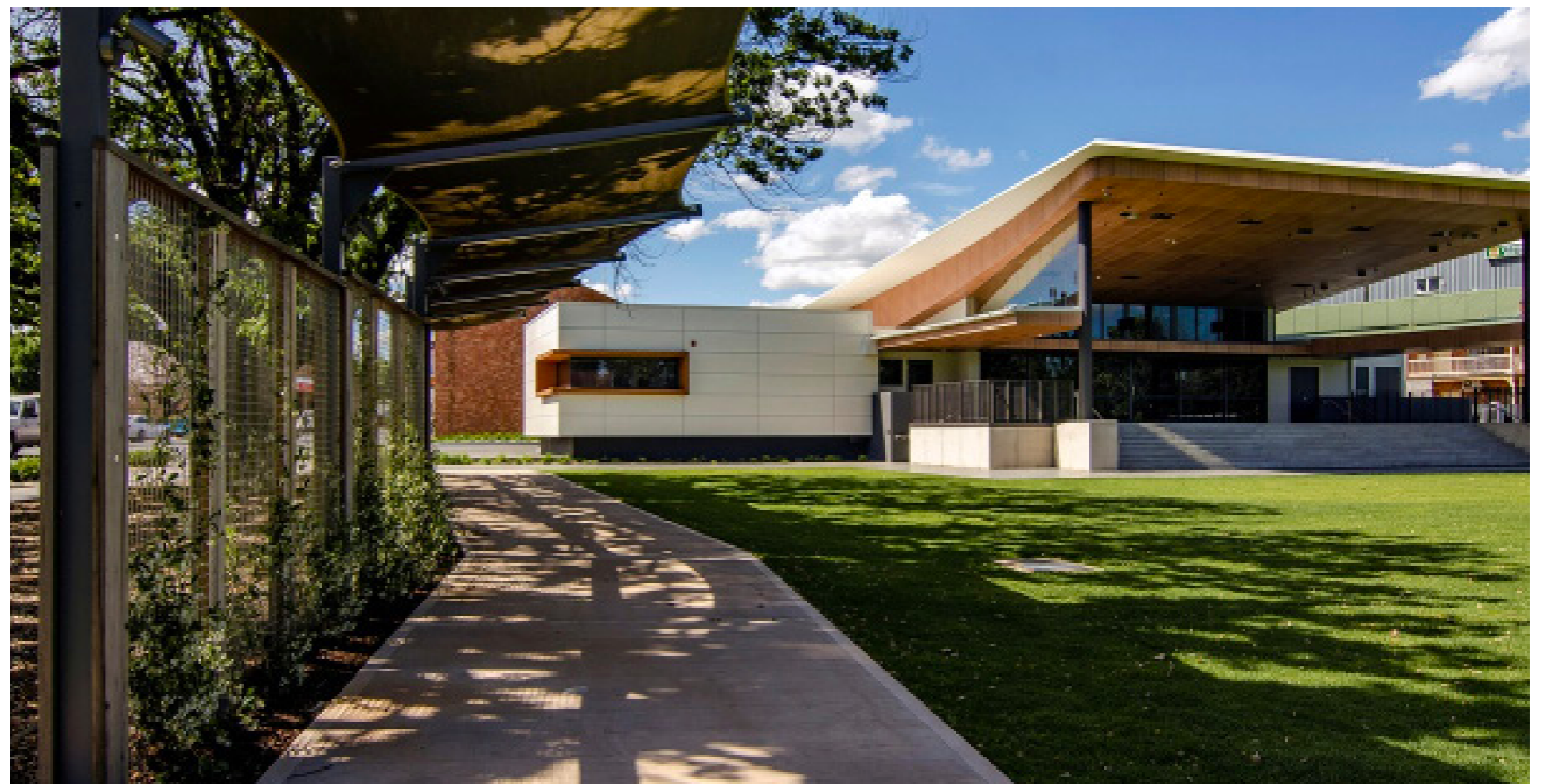
The recently completed Cooke Park Pavilion
