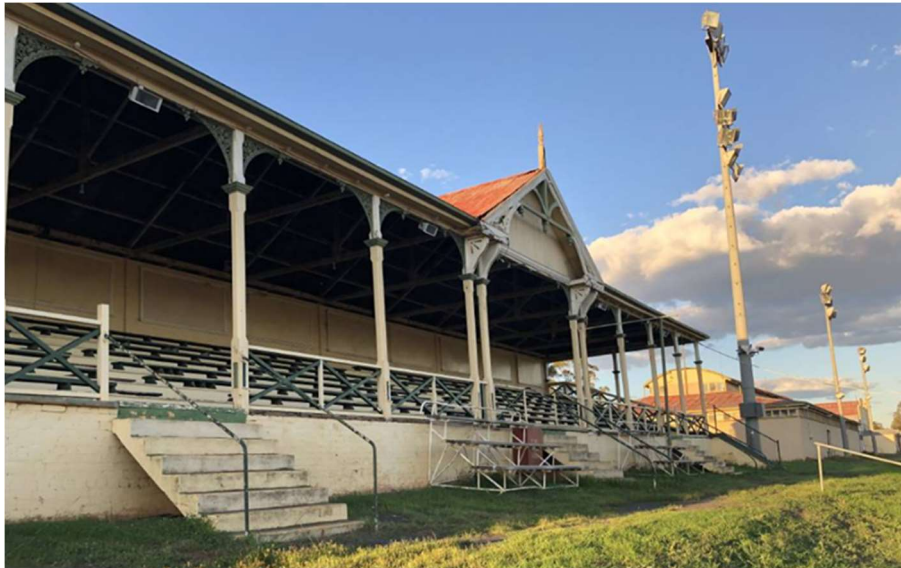
Grandstand building south side
